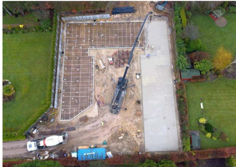
programme, completing our work in just four weeks and save the client the substantial associated costs of extensive excavation and concrete required for a piled beam scheme.
