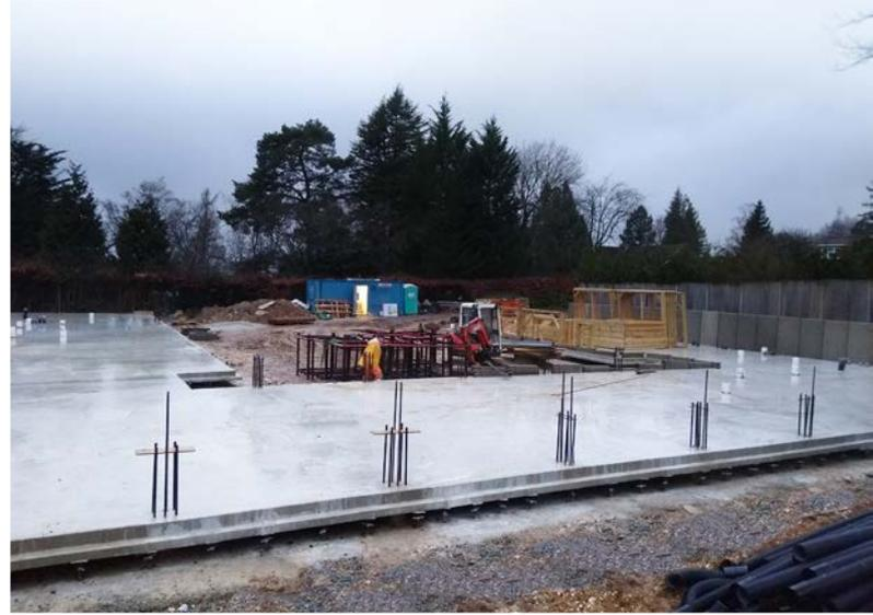
setting out points and levels to become unclear or lost. As we use a Concrete Working Surface (CWS), in lieu of a traditional granular piling mat, the groundworker was able to re-programme the installation until after piling was complete and work from the clean and stable platform provided by the CWS.
