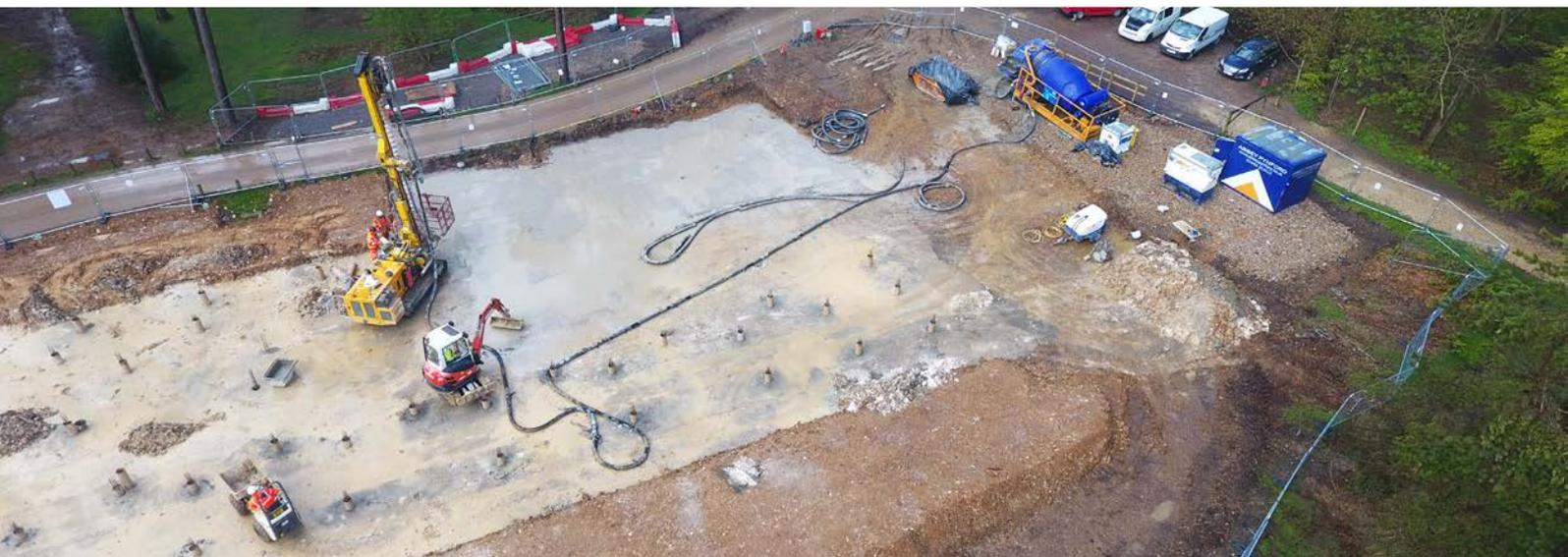
voided system allowed the superstructure to be isolated from future ground movement, ensuring the longevity of the structure from future ground movement.
